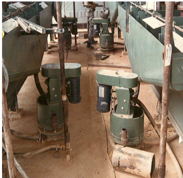
1" QPEC Vertical Sand Pumps being installed in Africa
